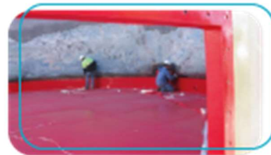
Piso Tanque - Concreto verde - HLT / EP-2 / Nukote ST 2.5mm
