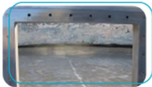
Piso Tanque - Concreto verde - HLT / EP-2 / Nukote ST 2.5mm
