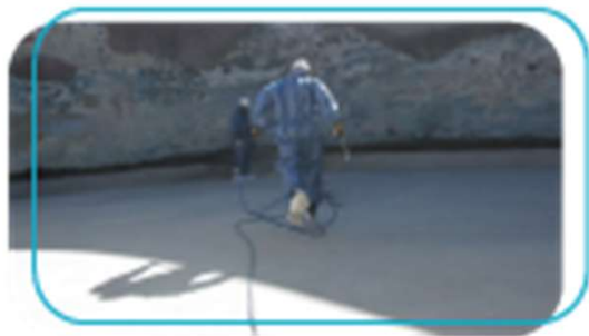
Piso Tanque - Concreto verde - HLT / EP-2 / Nukote ST 2.5mm
